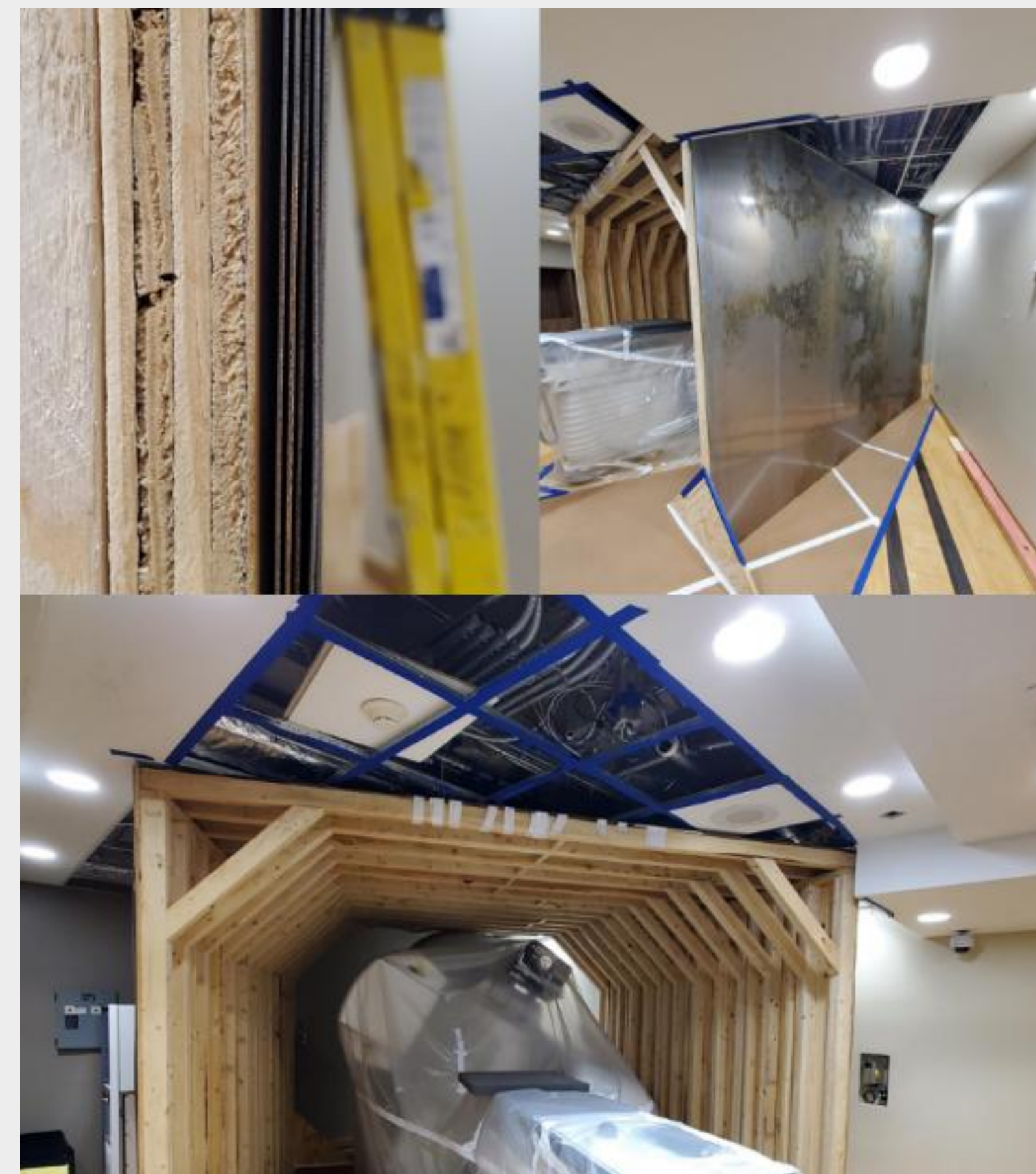
Figure 3: Photographs of the temporary (prototype) shielding enclosure. Top left: cross sectional view demonstrating layers of steel, plywood, and wooden frame assembly. Top right: Side view. Bottom: Front view.
